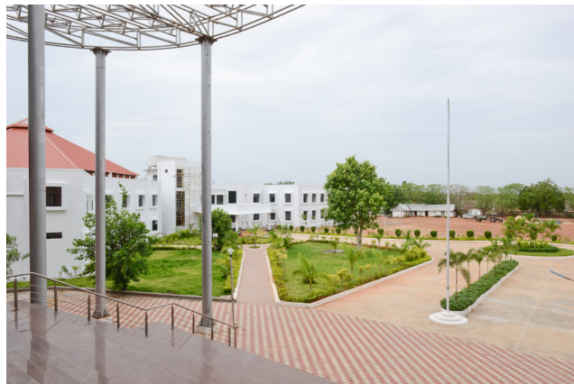
Completed Phase II Building – Academic Block 2012
