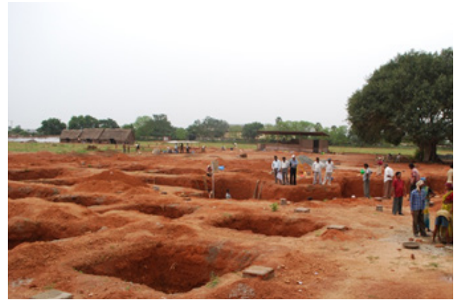
Foundation work for the New Building for IICPT – Phase 1 2008
