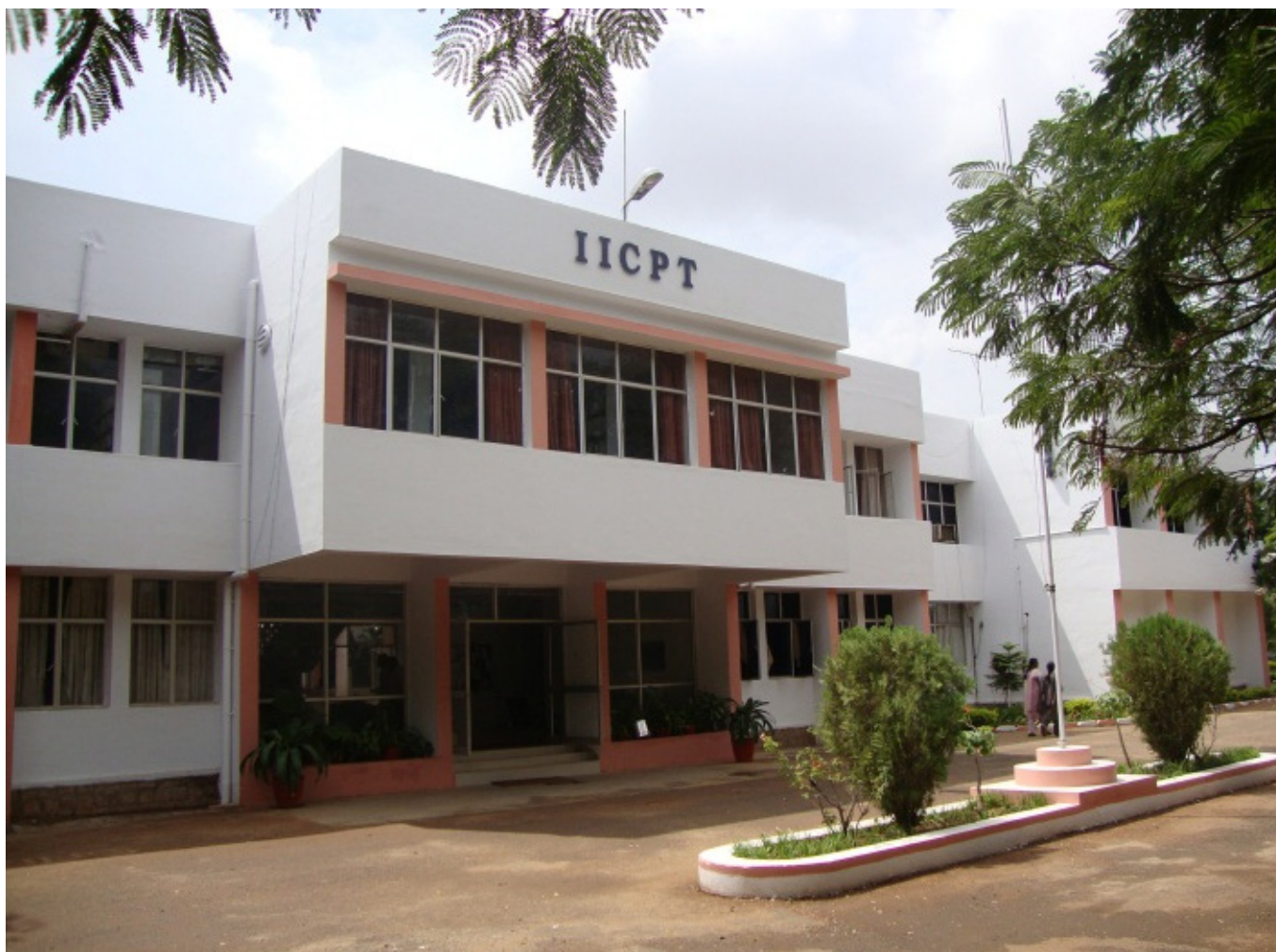
Indian Institute of Crop Processing Technology, Main building , 2008, Thanjavur-613005
