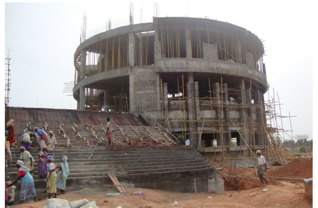
IICPT – New Building Work in Progress - Phase 1
