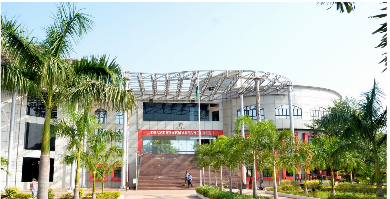
Completed Phase I - Dr. V. Subrahmanyam Block, IICPT
