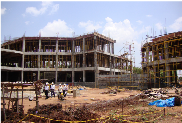
IICPT – New Building Work in Progress - Phase 1
